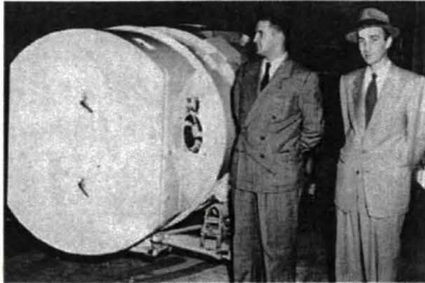
•Air-transportable dewar for 750 liters of liquid hydrogen developed by H.L. Johnston. ca. 1952. •First LN2 shielded vessel (77 K radiation shield).
