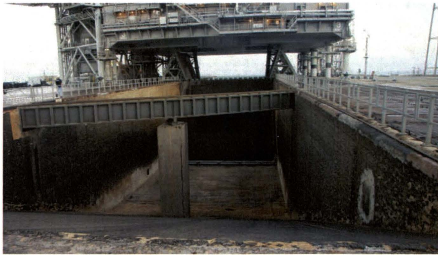
Figure 5. SSME Flame Trench
