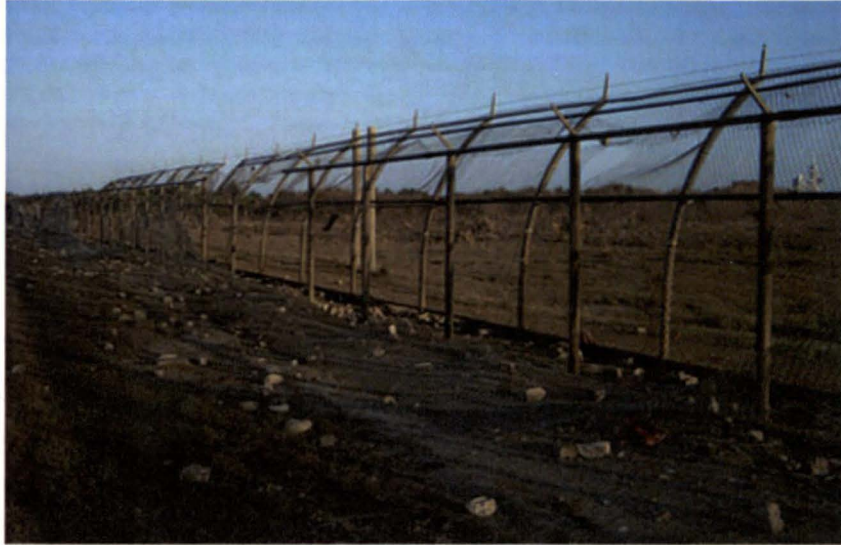
Figure 11. Refractory Concrete Bricks Around Fences
