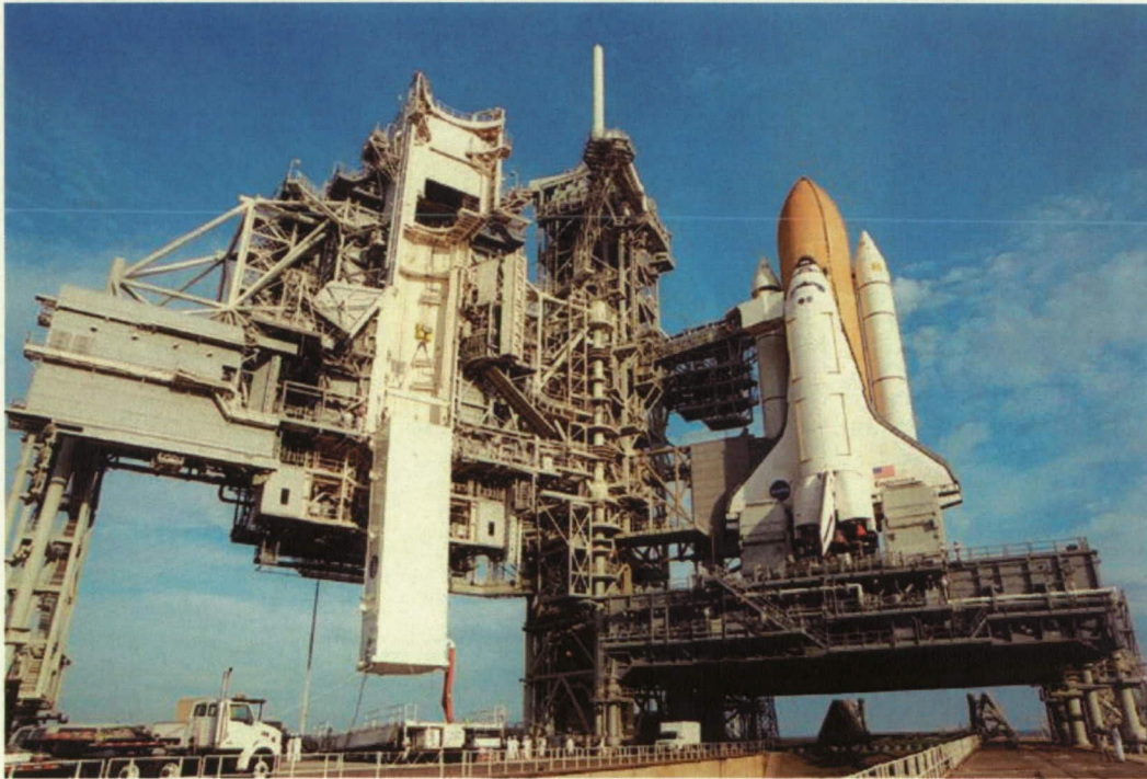
Figure 27: Payload Canister Lifted into PCR [NASA].
