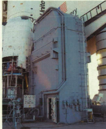
Figure 54: One of Two Shuttle Tail Service Masts [NASA]
