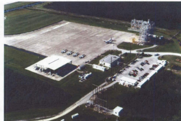
Low level aerial view of SLF of parking area
