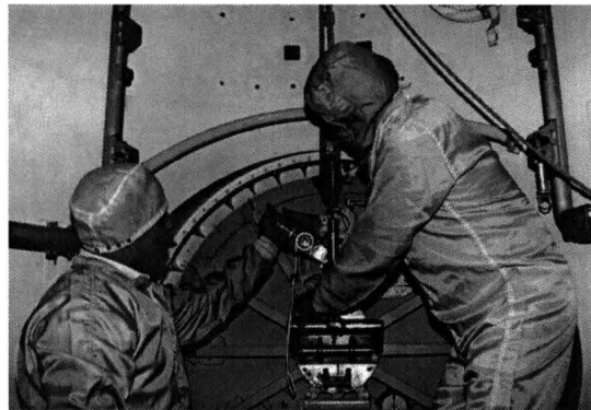
Figure 4: Engineers continue testing on the interior side of the outer airlock hatch to identify malfunctions. NASA Image
