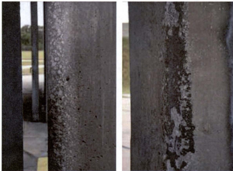
Figure 35. Damage to Side Flame Tunnel Support Columns
