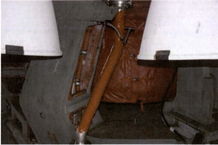
Figure 44. Ablative Coating on Tubing in Center of LC 17B Launch Deck
