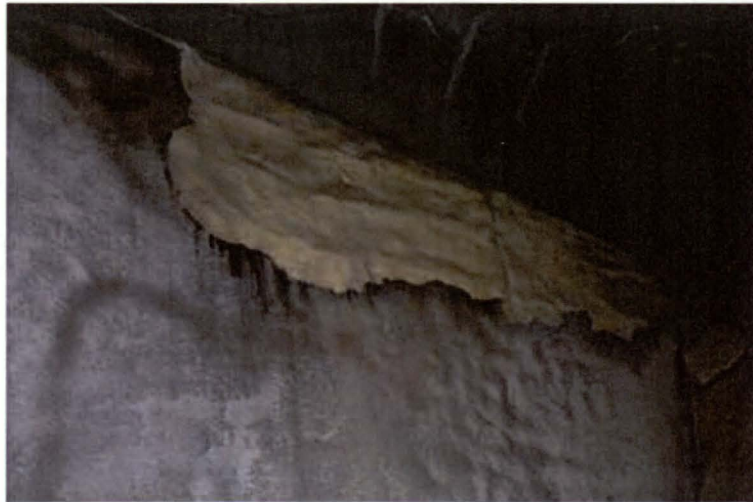
Figure 39. Martyte Patch on Flame Deflector Side Wall
