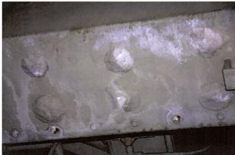
Figure 41. Martyte-Protected Bolt Heads
