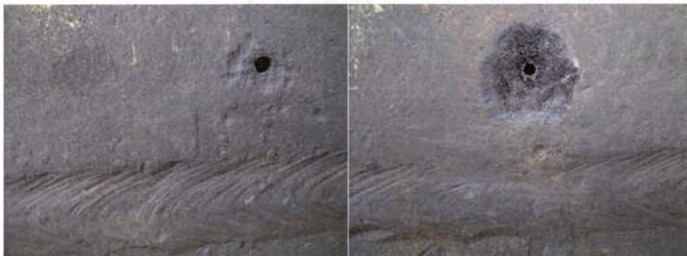
Figure 17. Drain Holes at the Base of the B-2 Flame Deflector
