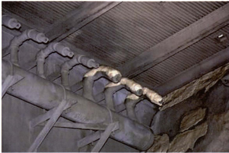
Figure 40. Martyte on Water Deluge System
