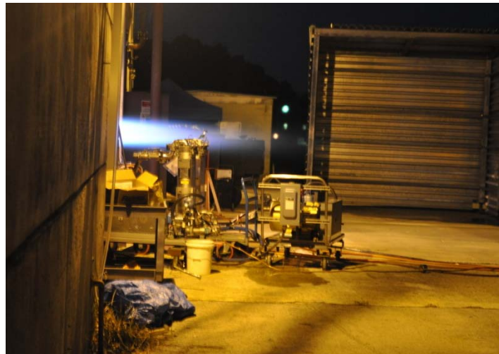
Afterburner Flame at Night
