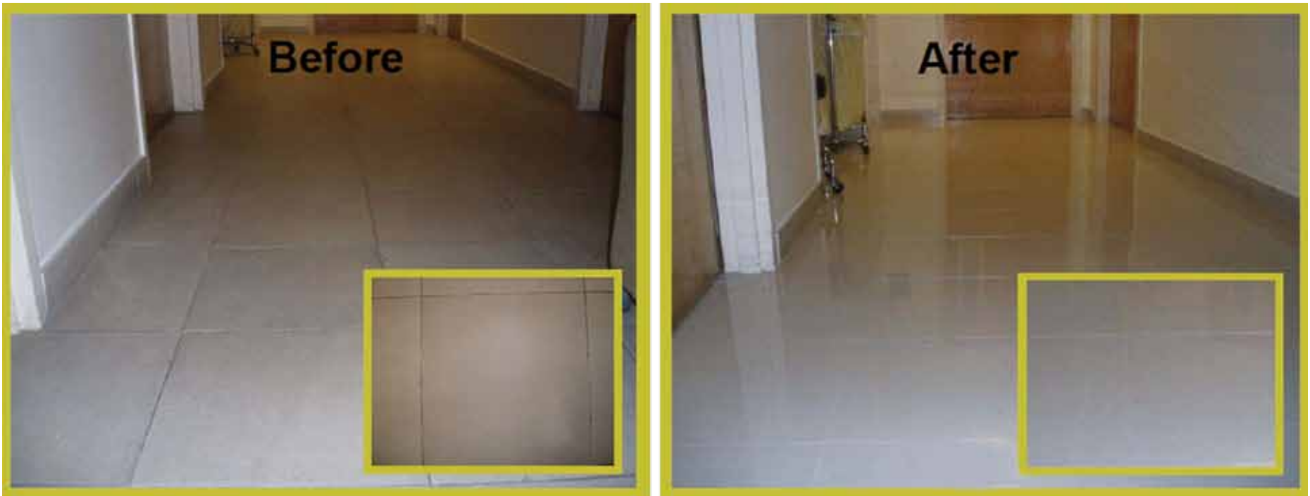
The tile floors of a hospital in Miami, Florida, are shown before and after being coated with Adsil Corporation's MicroGuard Clear Treatment System. According to Adsil, the coating will lessen the maintenance of the floors and improve the floors' appearance. Adsil's coatings are derived from John B. Schutt's work at Goddard Space Flight Center on durable coatings for spacecraft.
