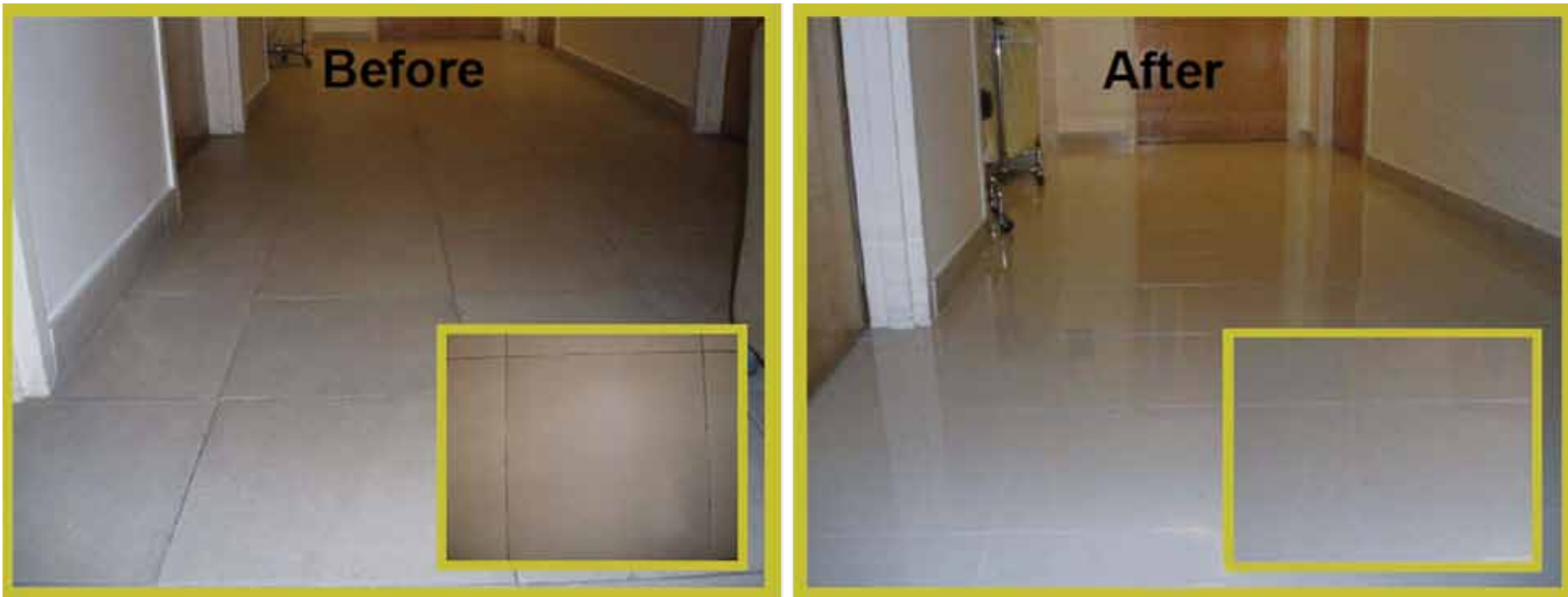
The tile floors of a hospital in Miami, Florida, are shown before and after being coated with Adsil Corporation's MicroGuard Clear Treatment System. According to Adsil, the coating will lessen the maintenance of the floors and improve the floors' appearance. Adsil's coatings are derived from John B. Schutt's work at Goddard Space Flight Center on durable coatings for spacecraft.
