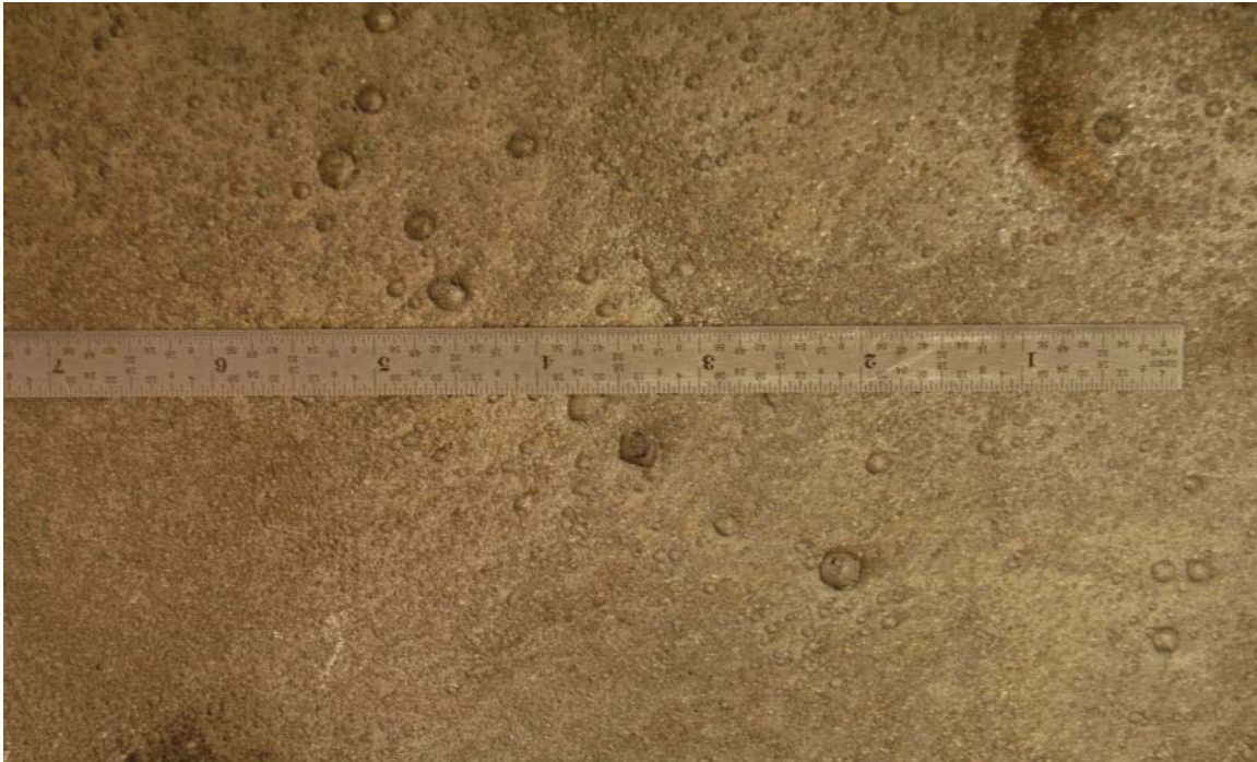
Figure 7.1-11. Backside of Impact Plate 1907 (this plate shows extensive pitting across most of the plate (~15-inch radius of debris damage); a few larger pits, seen as an arc across the photo, are actually minor penetrations in the form of short cracks)
