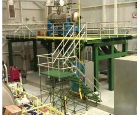
Chamber in Place on Platform
