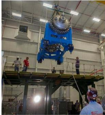
Chamber Lifted into Place
