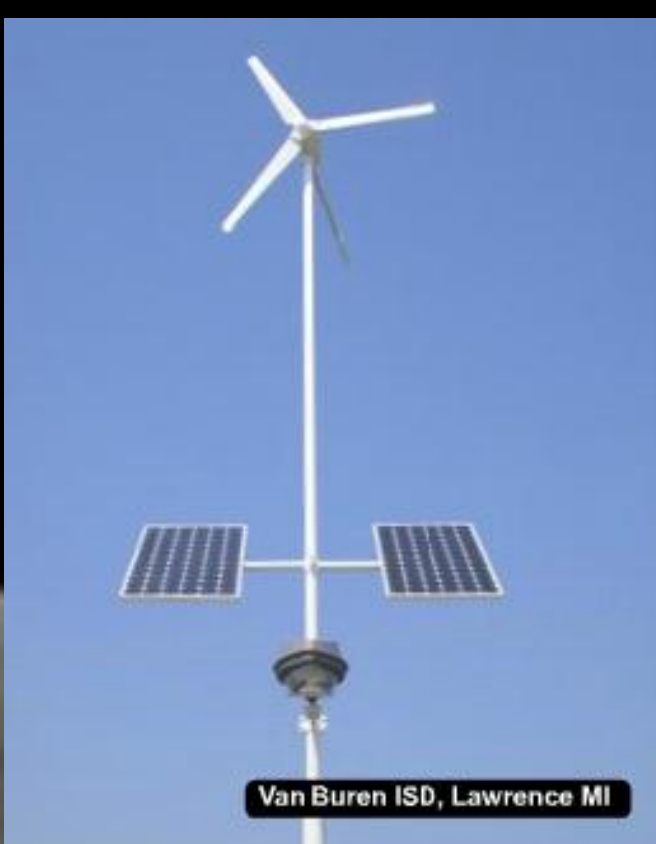
Wind/Solar Hybrid lights previously installed at JSC
