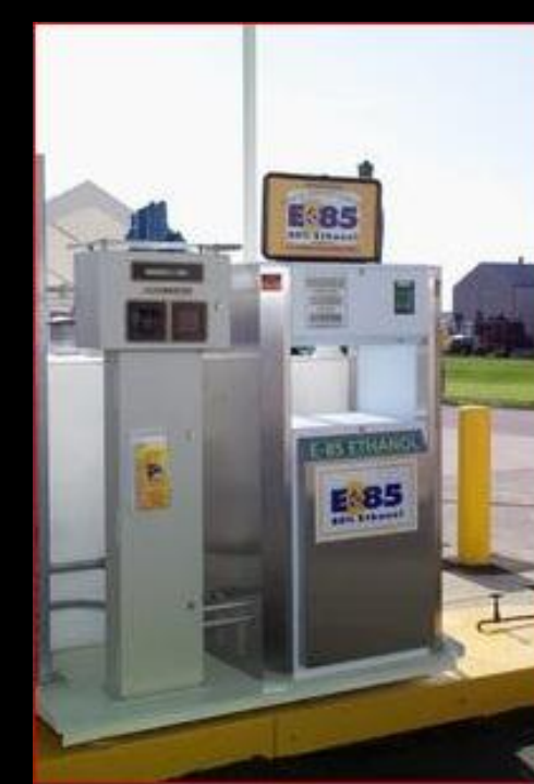
E-85 Fueling Station
