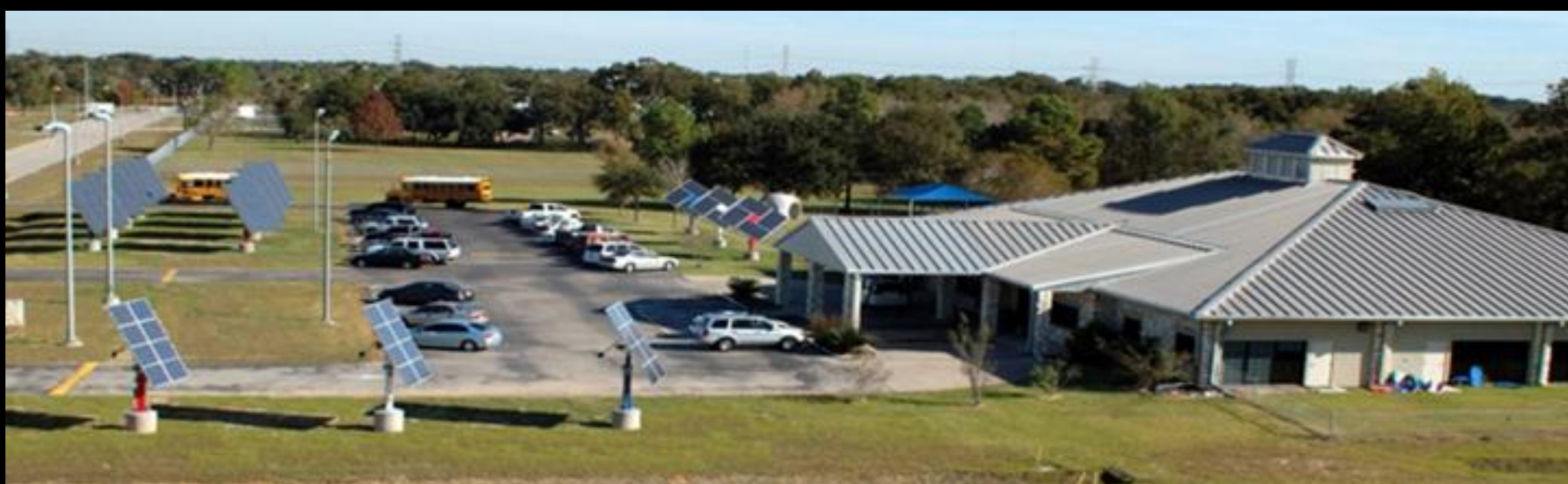
Child Care Center Renewable Energy System
