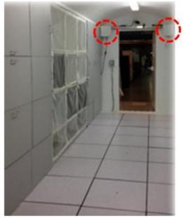
Figure 6. Red circles mark antennas for the sparse area reader.
