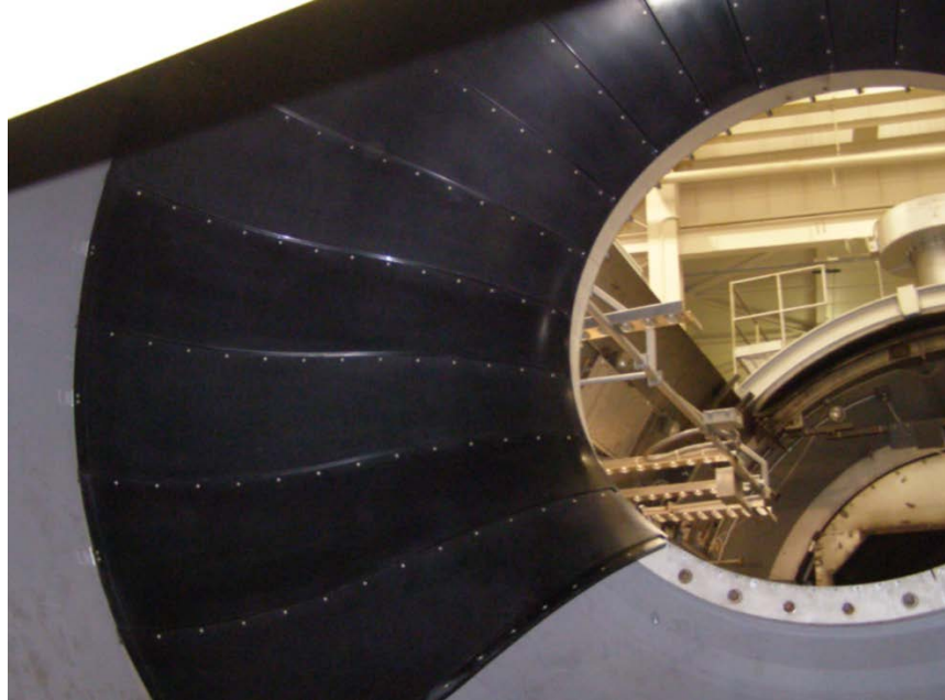
Figure 7. Carbon fiber transition panel installation.
