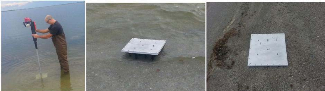
Figure 11. Post-hole driver inserting blanket and blanket in various stages of insertion
