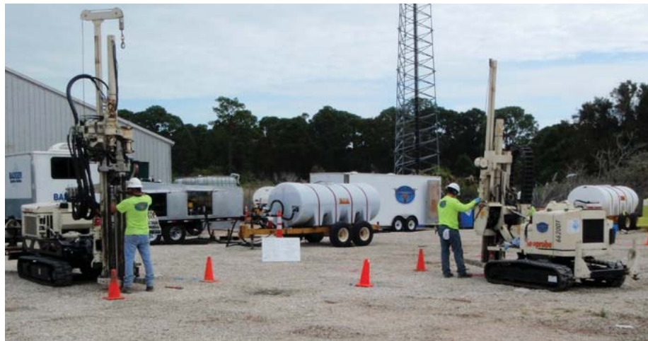
Technicians inject EZVI into the ground in two locations.
