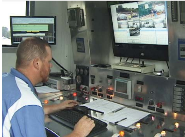
A technician monitors the injection process.
