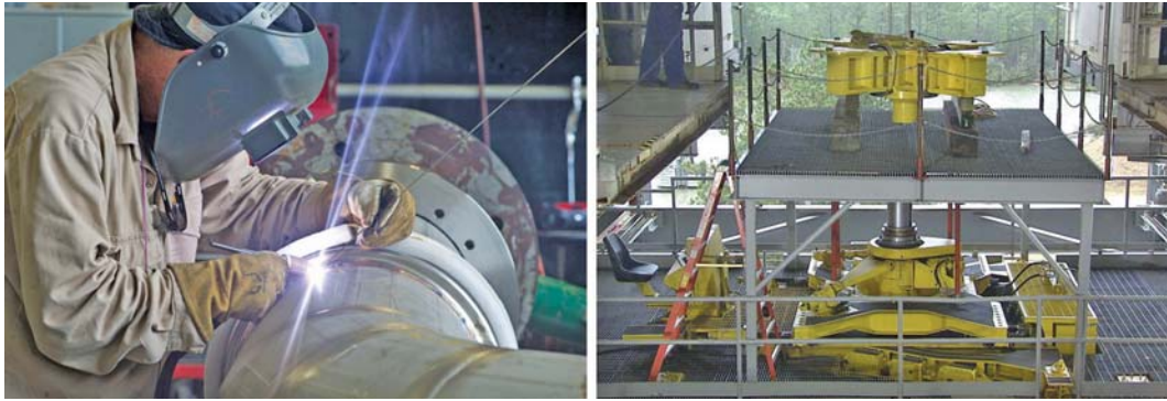
Fig. V: Renovating the SSC A-1 test stand (left) and RS-25 thrust frame adapter (right)
