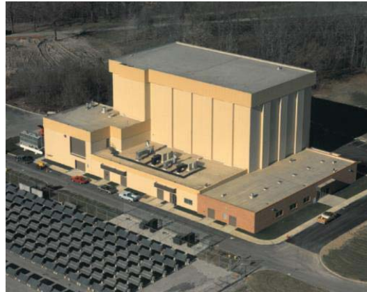
Figure 4. GRC Power Systems Facility (PSF)
