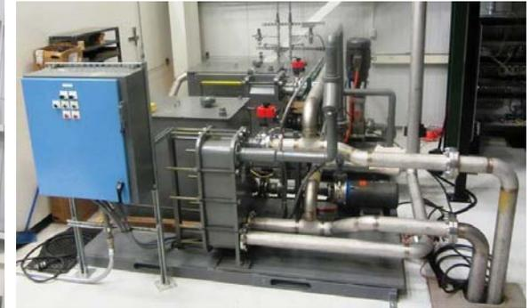
New Cooling Water System now provides 2 separate systems that cool induction coil and power feedthrough, induction heater and H<sub>2</sub>N<sub>2</sub> mixer respectively
