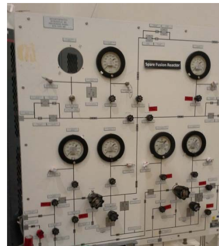
Figure 5 - Pressure regulation panel for HMA testing.
