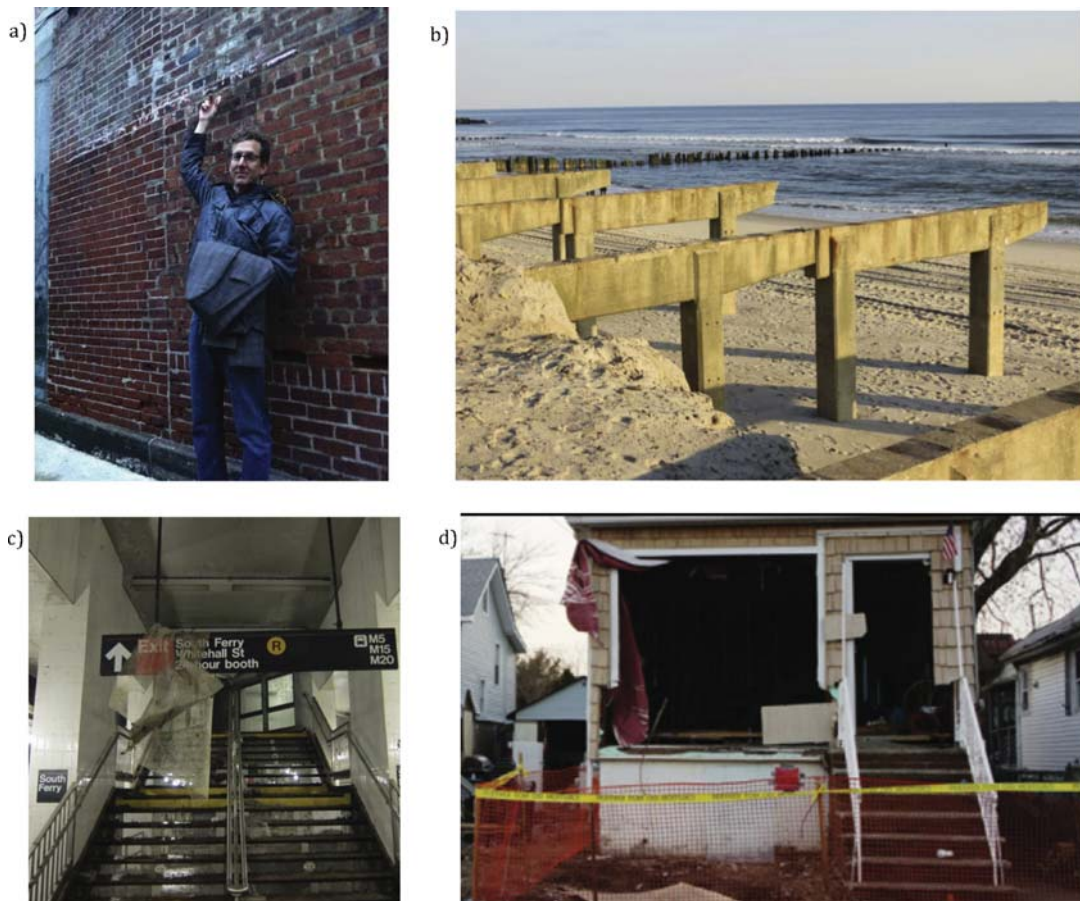
Fig. 3. Impacts of Hurricane Sandy in New York City: (a) High water mark at South Street Seaport, Manhattan (Phillip Orton, Stevens Institute of Technology). (b) Concrete support beams at the boardwalk destroyed in Rockaway Park, Queens (Gary Monitz, Columbia University). (c) Damage at South Ferry subway station in Manhattan (Daniel Bader, Columbia University). (d) Damaged home in Staten Island (Somayya Ali, Columbia University).
