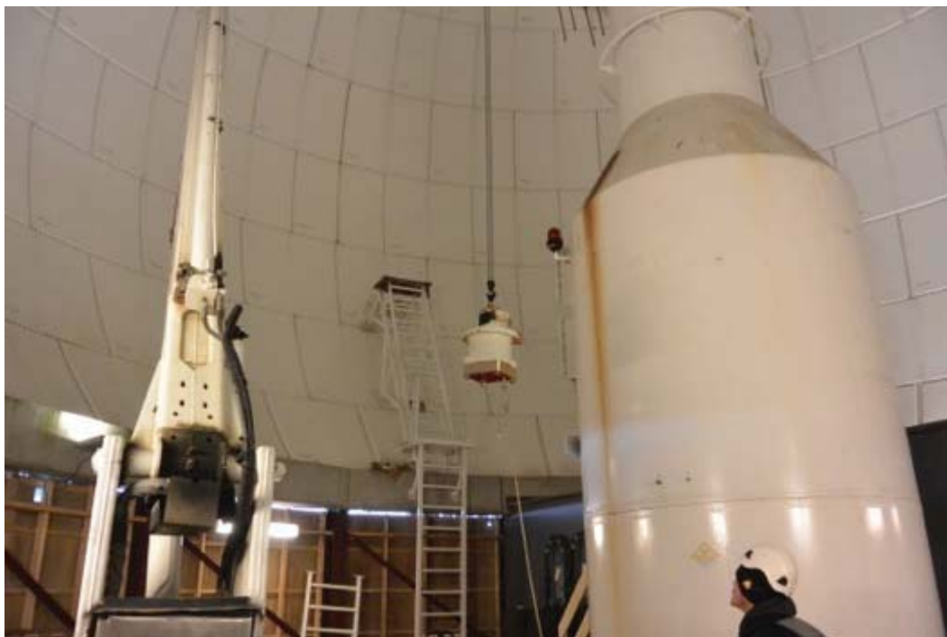
Removal of Elevation gear and motor
