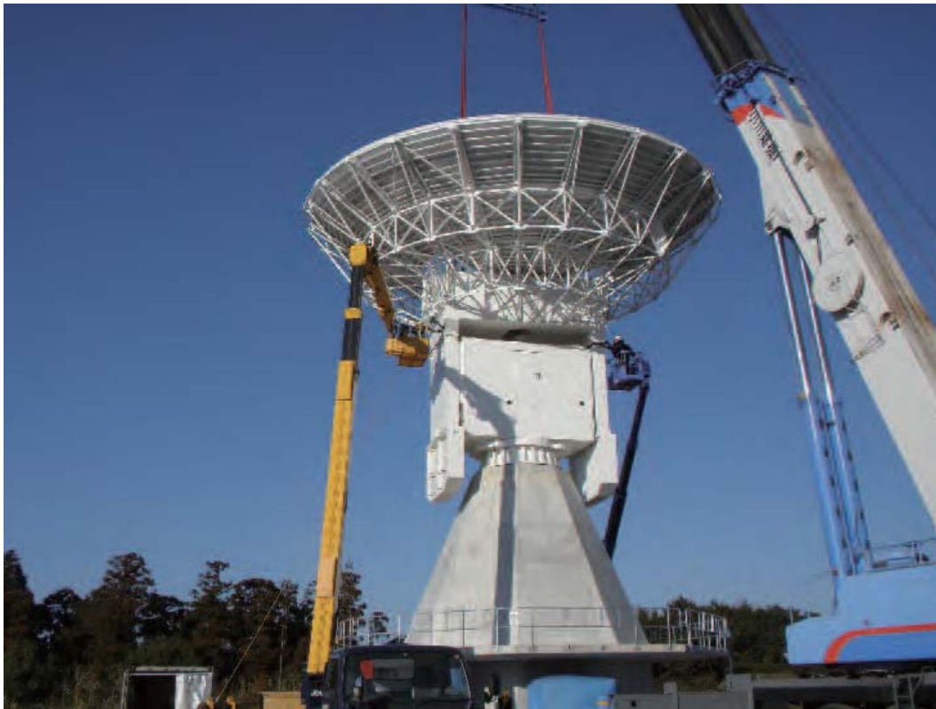
Fig. 5 Construction of the antenna.
