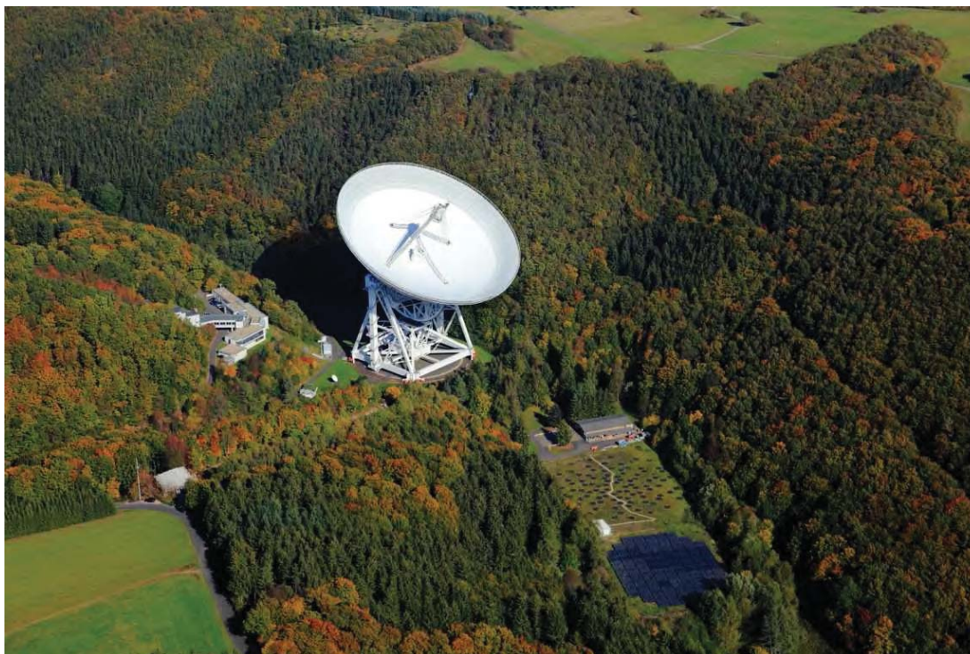
Fig. 1 Aerial image of the Effelsberg radio observatory. Shown are the 100-m Effelsberg antenna and the institute building. Effelsberg hosts also a station of the European Low Frequency Array (LOFAR), seen in the lower part of the picture.
