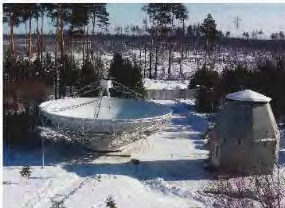
Fig. 6 Main reflector 13.2-m and antenna tower.
