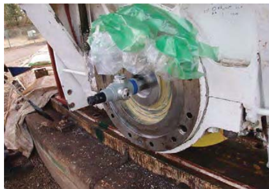
Fig. 2 Installation work of new azimuth wheel.
