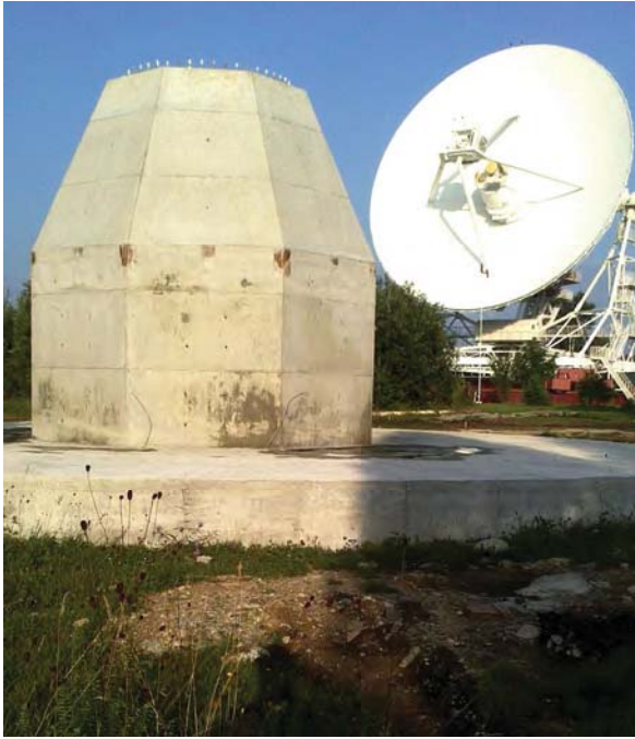
Fig. 4 Antenna tower for the 13.2-m dish and RT-32 at Zelenchukskaya observatory.
