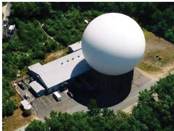
Fig. 1 The radome of the Westford antenna.
