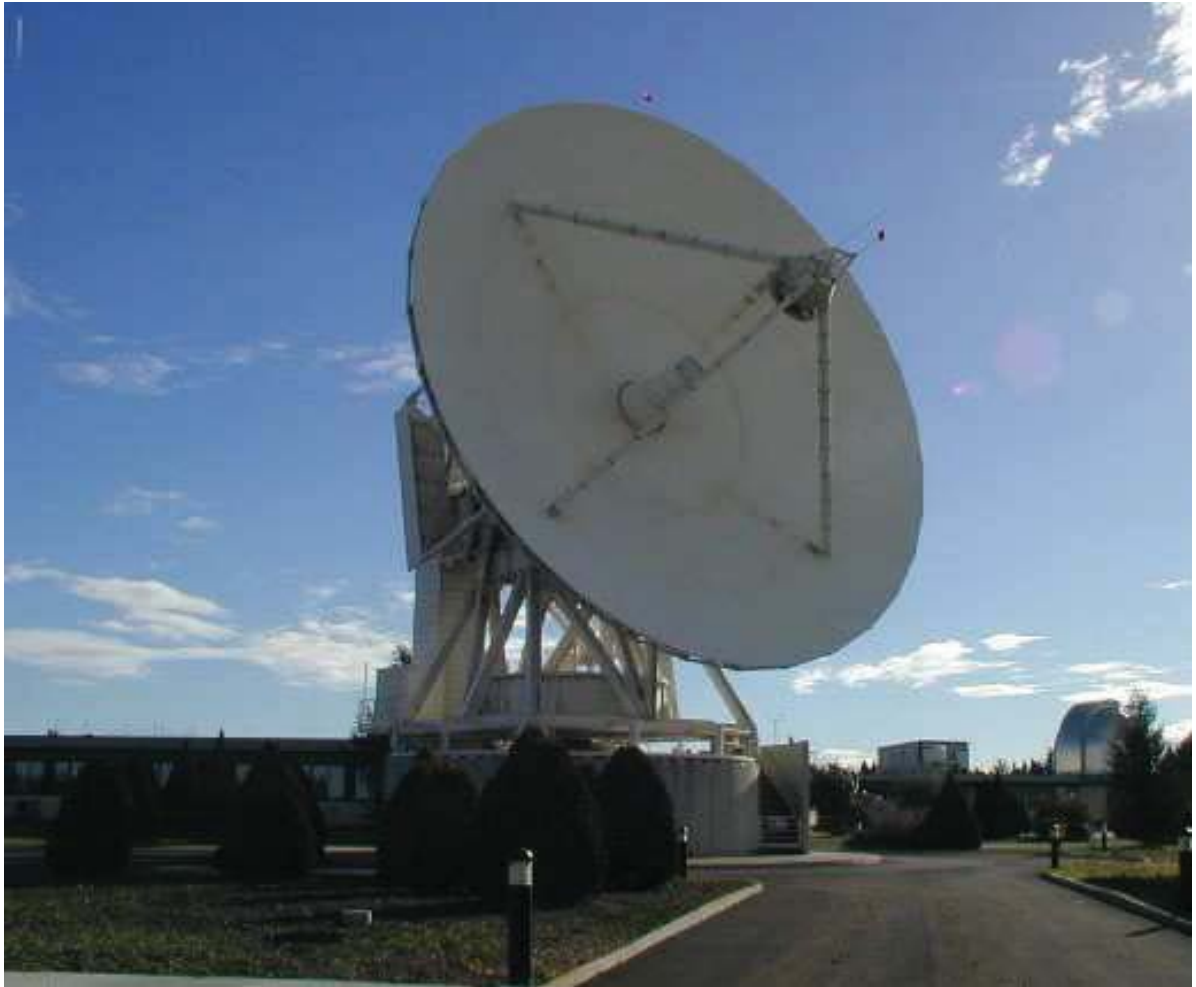
Fig. 1 VLBI antenna and MLRO dome.
