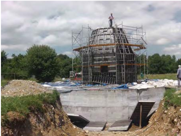
Fig. 4 Autumn 2013, building in progress.
