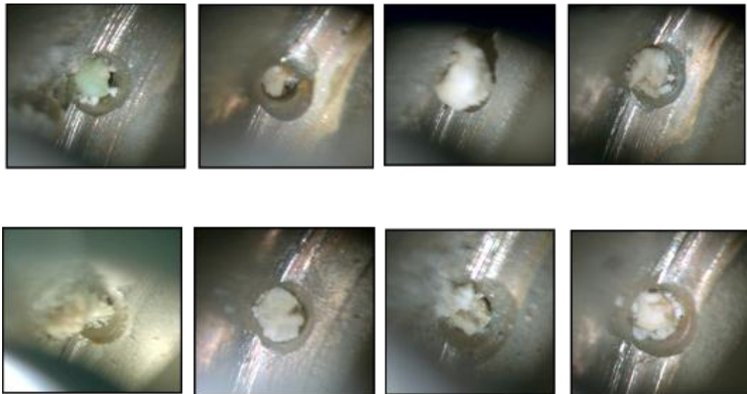
Figure 3. Blocked water separator drum holes.
