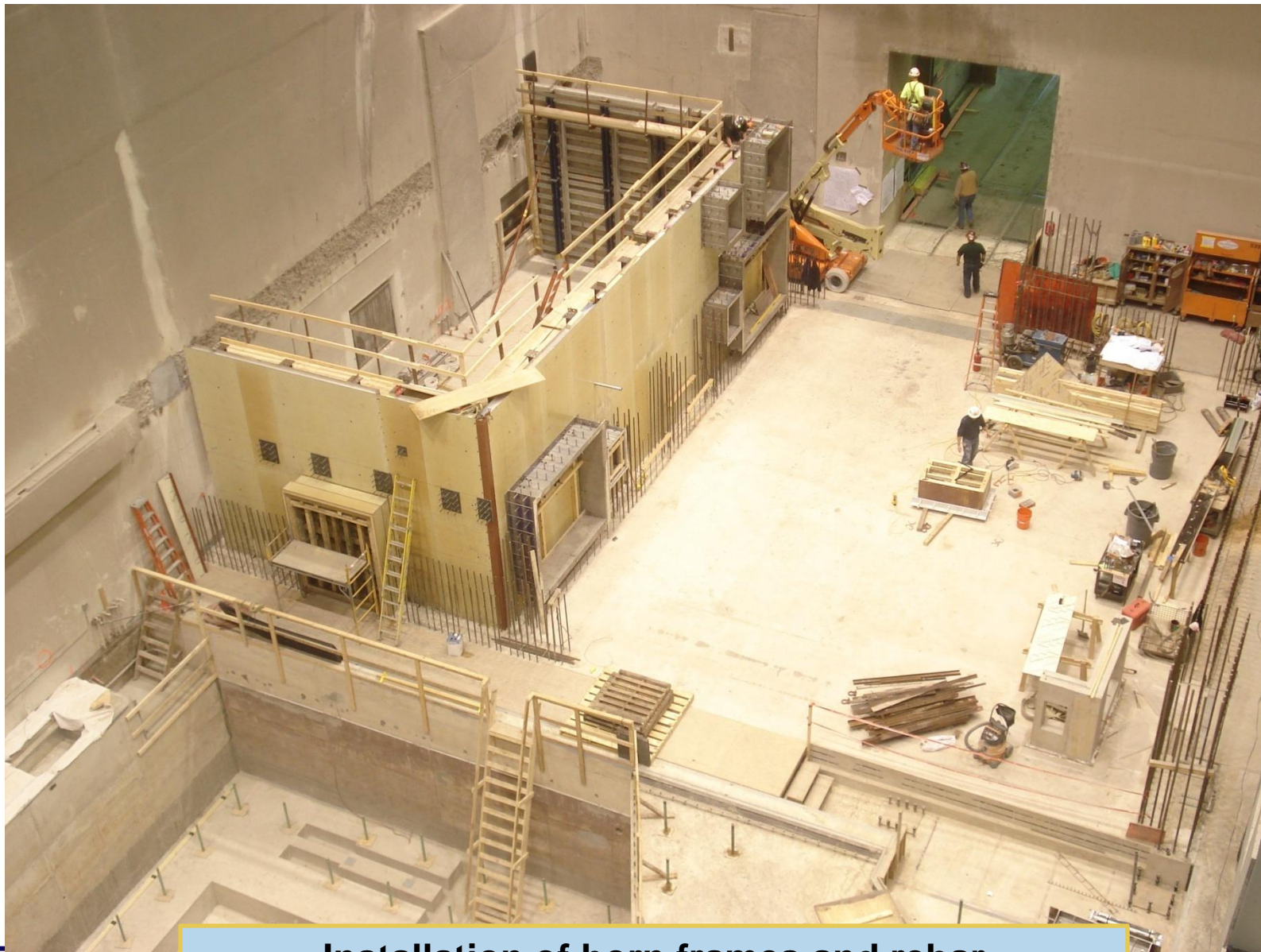
Installation of horn frames and rebar
