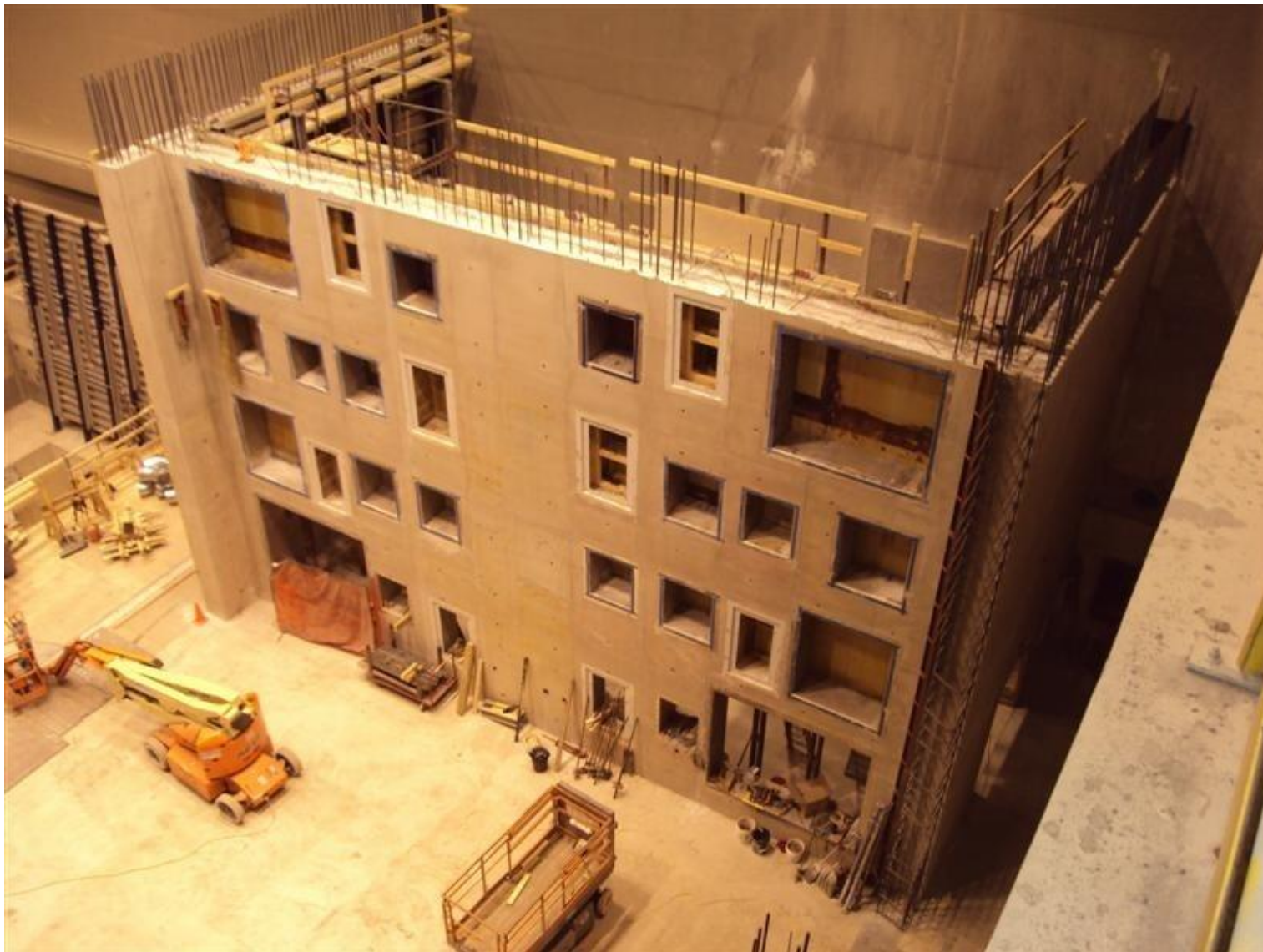
Concrete pour #2 completed with forms removed
