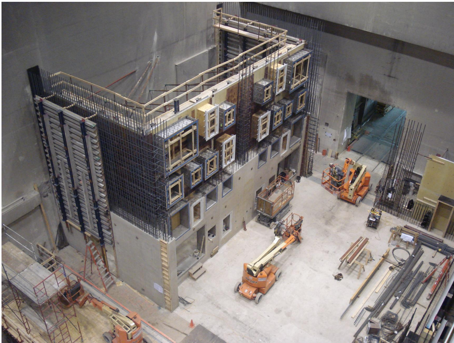
Horn wall level 2 horn frame and rebar installation
