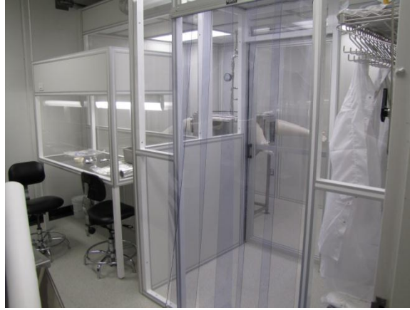
Figure 26: ISO class 5 cleanroom with ACG.
