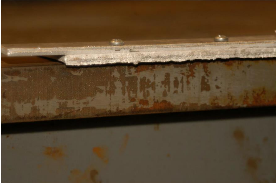
LSC Plate Close-up, Post-Test, Test T01
