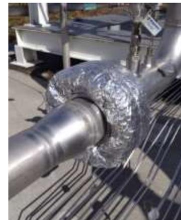
Basic installation sequence of LCX on a piping flange assembly (bolted joint).
