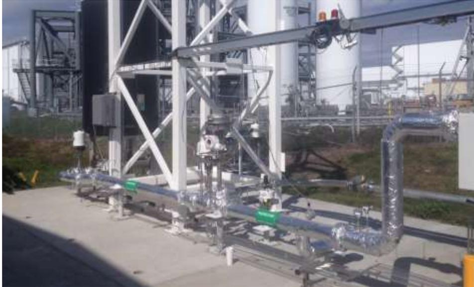
Completed LCX installation on the Rapid Propellant Loading System at Kennedy Space Center, showing a combination of piping, valves, pipe supports, and flanges.
