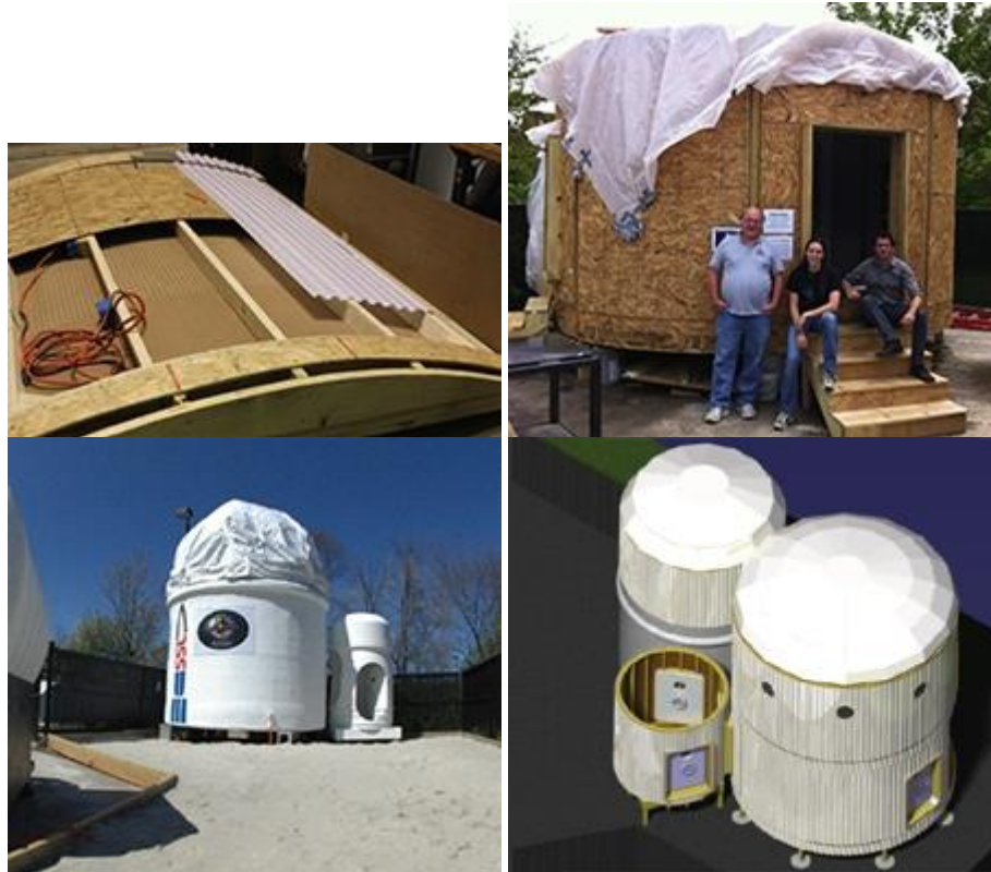
Figure 5: From top left, clockwise: A wall of the vertical habitat prototype by University of Maryland students; Early prototype built for living simulations at the University of Maryland, College Park; Concept for stacking of multiple vertically oriented modules; Prototype built for living simulations at the University of Maryland, College Park. (Credit: University of Maryland)
