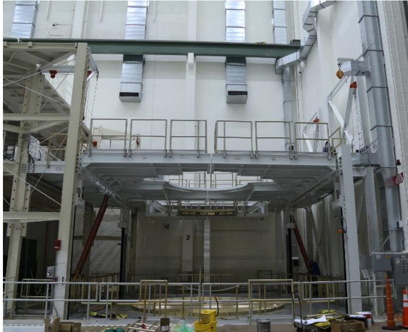
Figure 4: FAST Cell Just After Structural Completion
