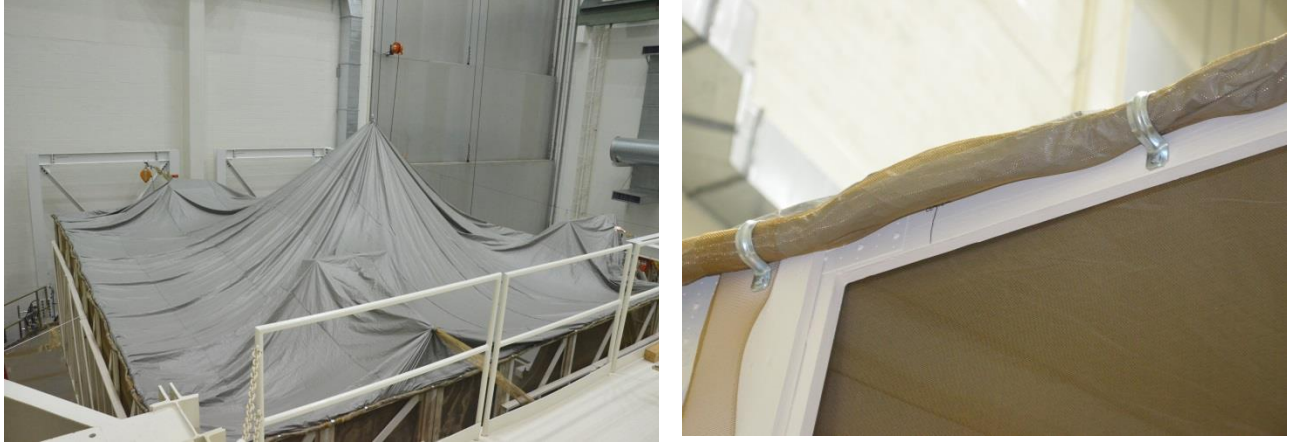
Figure 19: RF Fabric Roof in Place and Held with Pipe Clamps
