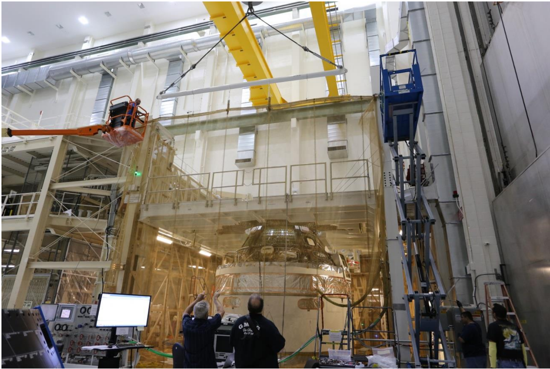
Figure 17: Front Curtain Closeout Being Craned into Place
