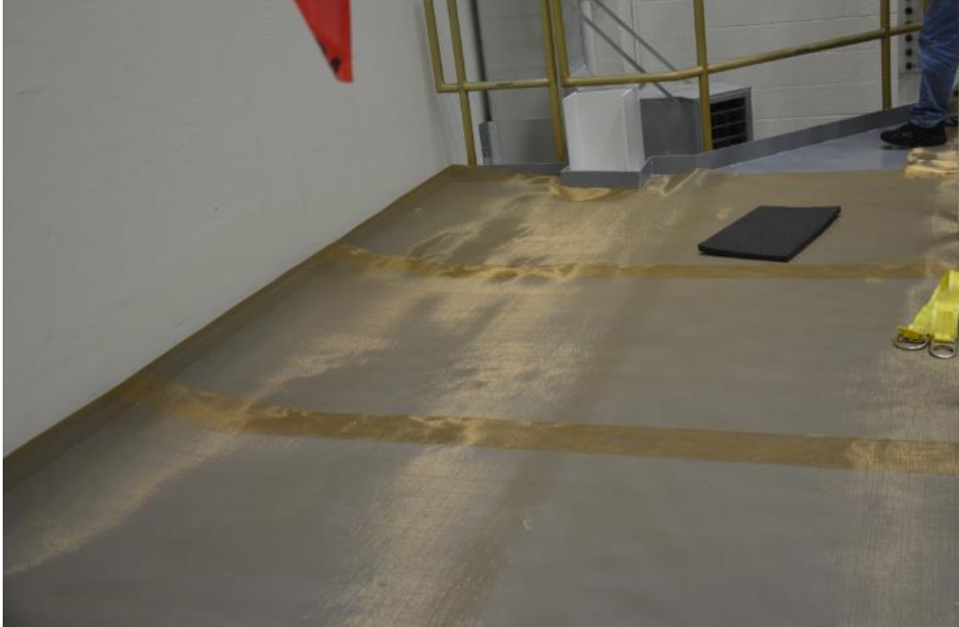
Figure 11: Screen-Wrapped Platform – from Above
