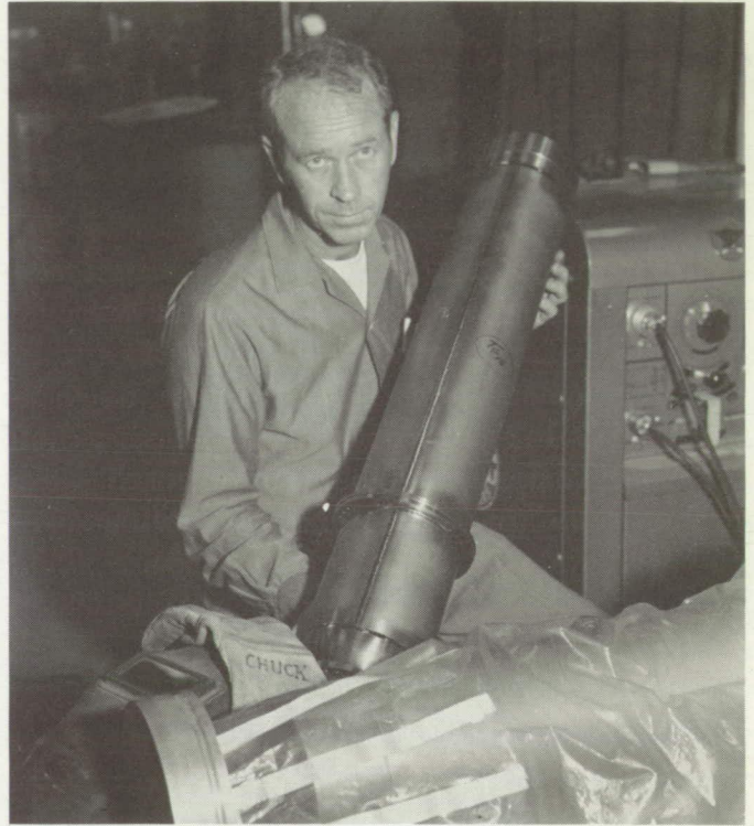
Fig. 4. Completed Weldment of Titanium-Alloy Motor Case
