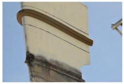
Figure 8.—Blade with shape charge around full circumference.
