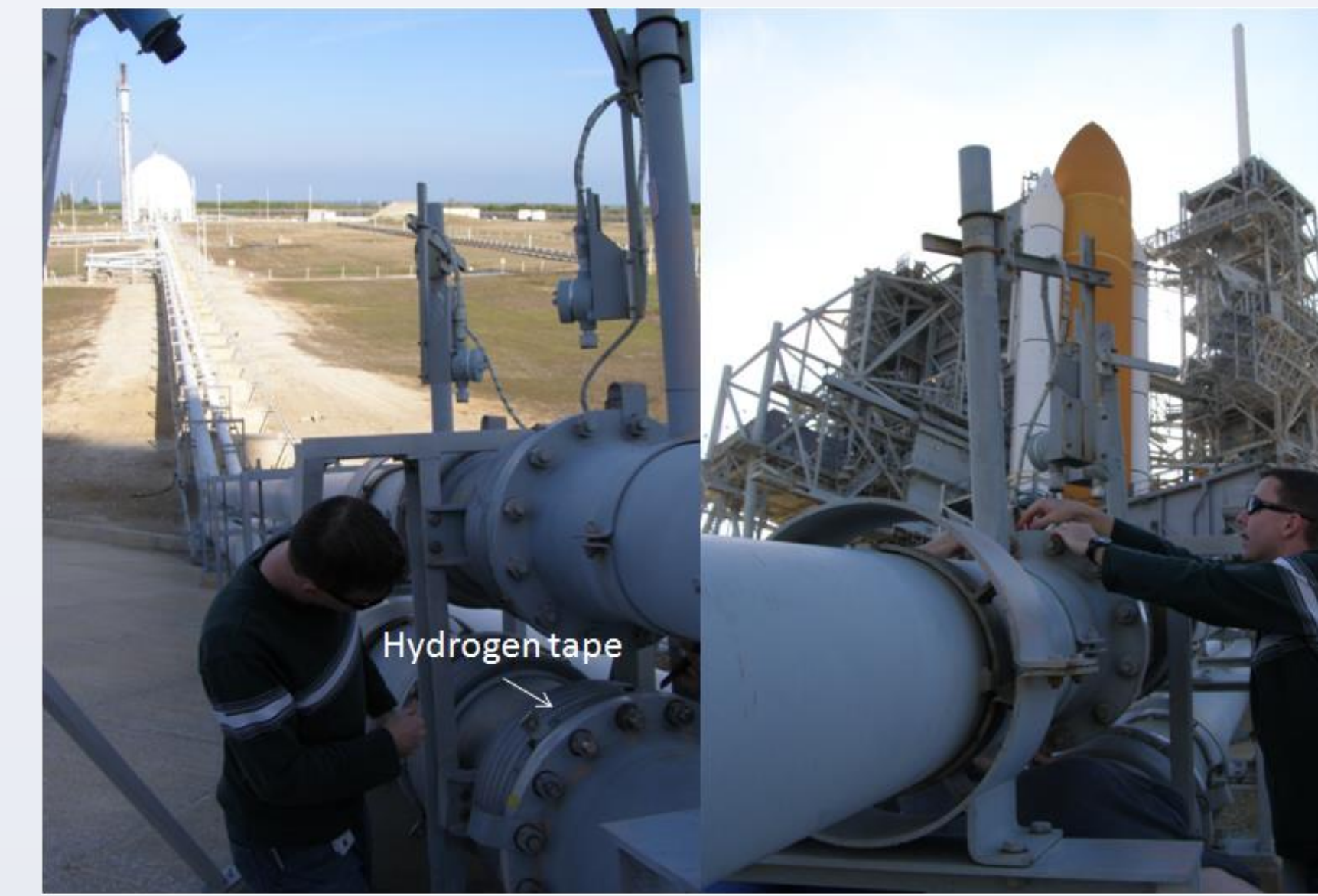
Deployment of tape for cross country lines during STS-130.
