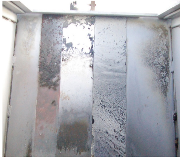
Figure 3. Ablative coatings inside the steel flame trench after 12 Morpheus free flight launches.
