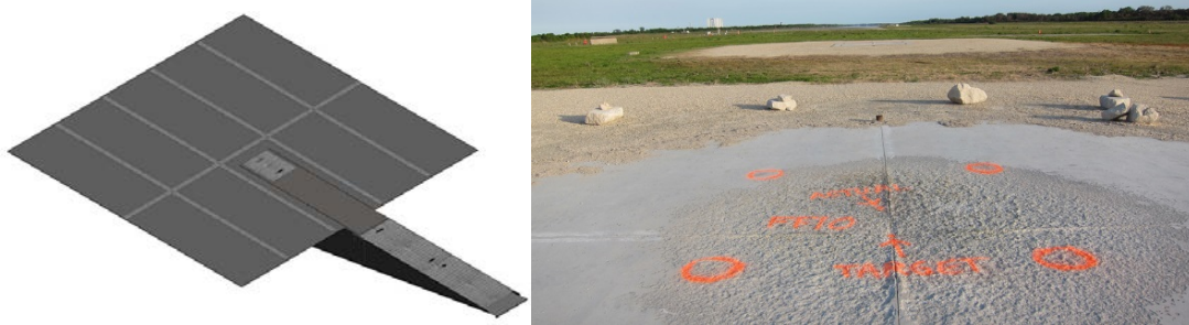
Figure 1. (Left) Schematic of a transportable modular steel launch/landing pad with attached flame trench. (Right) Landing pad at KSC showing cumulative spalling of concrete produced during the descent and landing of the Morpheus vehicle after free flight #10.
