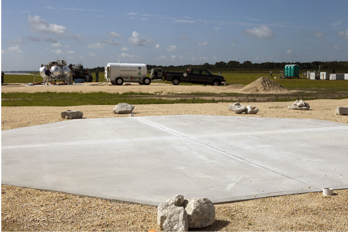
Figure 4. The original concrete landing pad used for descent and landing of the Morpheus lander.
