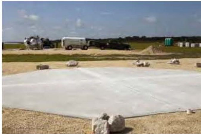
Original condition of concrete landing pad used during descent and landing of the Morpheus lander
