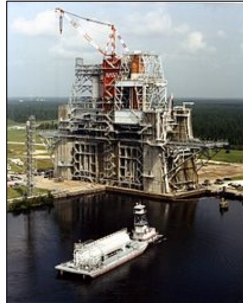
Figure 3 SSC B-Complex Test Facilities with propellant delivery barge in foreground
