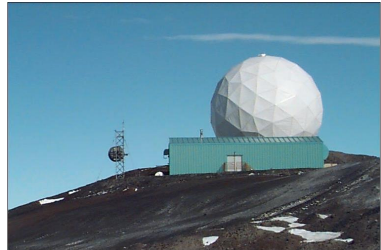
NEN McMurdo Ground Station
