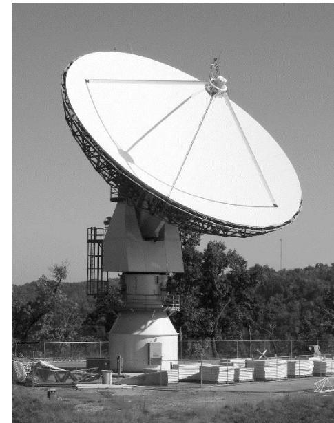
Morehead State University Space Science Center 21-M Ground Station, Morehead, KY
