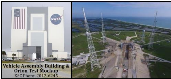
Figure 4: Launch Site Work Environment
