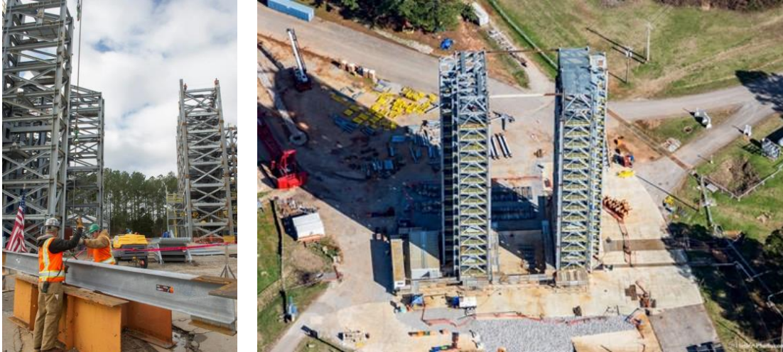
Figure.V: LOX (left) and LH2 (right) test stands under construction at MSFC
