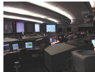
2 Operational Control Centers
