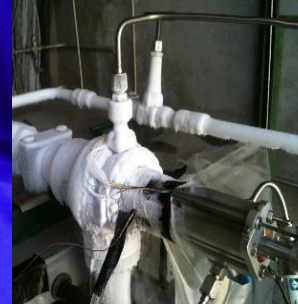
Main Fuel Valve Cryo Test
