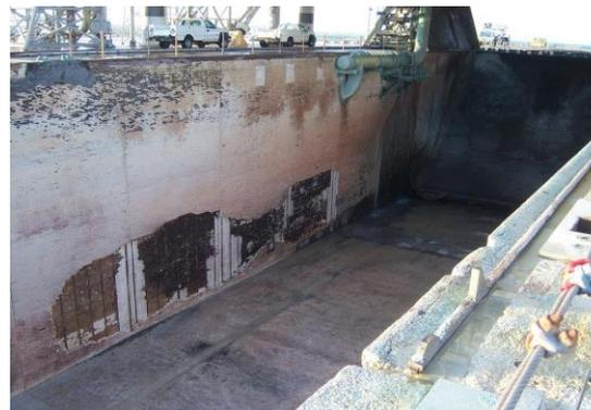
Launch Pad Flame Trench Damage
