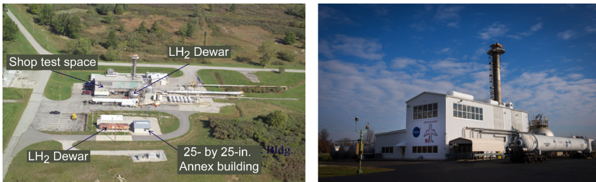
Figure 1.—Exterior of NASA Electric Aircraft Test bed (NEAT). LH 2 , liquid hydrogen.
