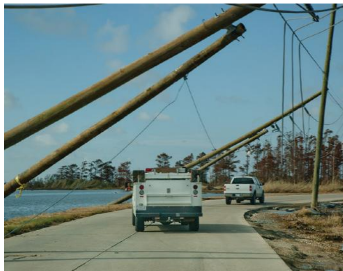
Power lines damaged by Hurricane Isaac's wind and surge in Plaquemines Parish, Louisiana, September 3, 2012.
