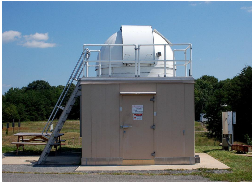
Figure 3-2: Front of NGSLR Shelter and Dome
