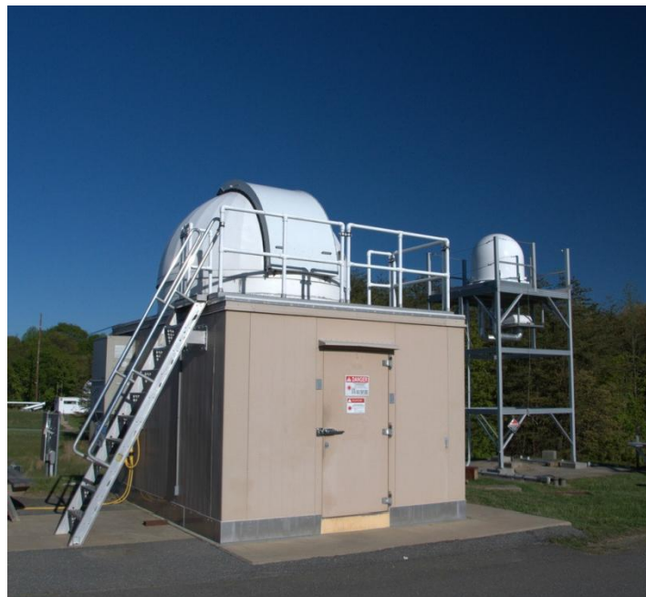
Figure 3-18: The NGSLR shelter (left) with the LHRS tower on the right
