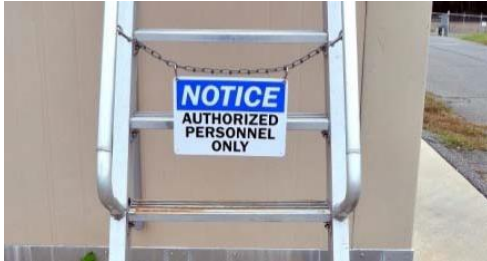
Figure 3-24: Stairway chain and warning sign
