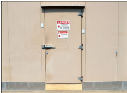
Figure 3-3: Locking handle and posted warning signs on entrance door
