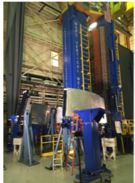
Figure 8. Welding of the Orion Stage Adapter at Marshall Space Flight Center.
