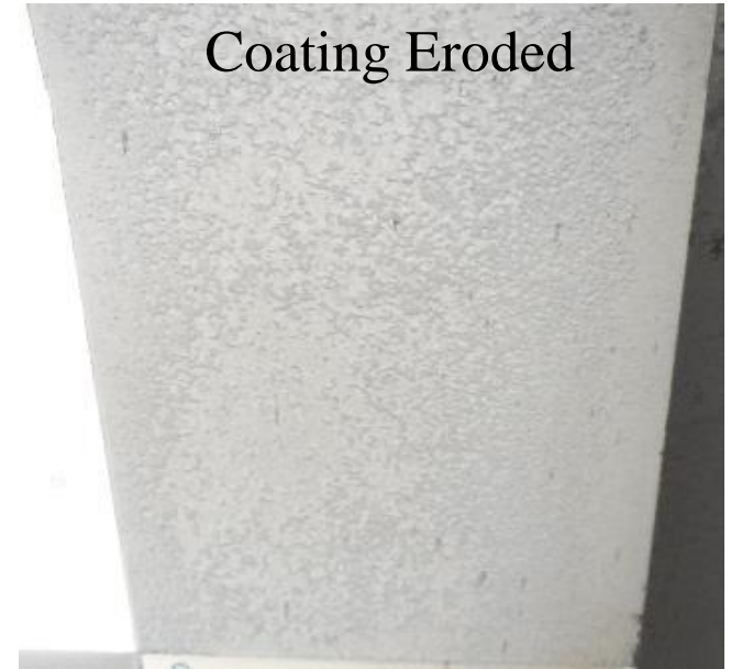
Discoloration / Signs of Coating Erosion
