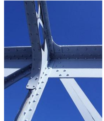
Indication of hidden corrosion by color change
