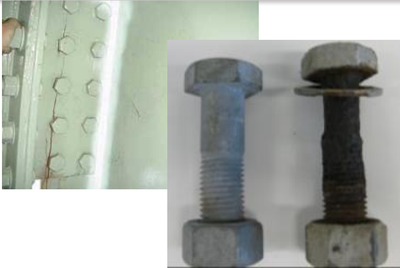
Enclosed / Inaccessible Areas
