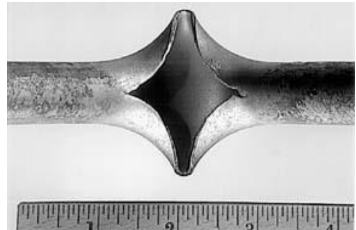
SS 304 tubing split caused by pitting
